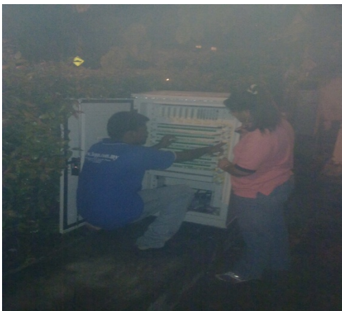
7. Finalizing splitters cable arrangement
