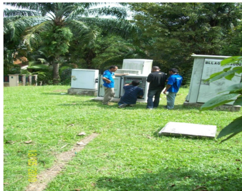
5. Finalizing adapters installation
