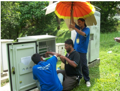
4. Installing adapters
