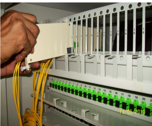
7. Installing splitters
