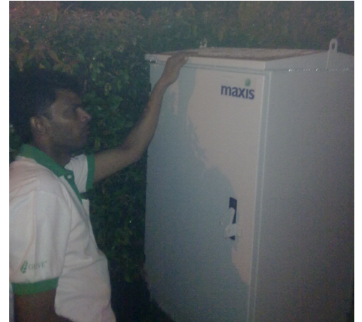
9. Complete installing FDC
