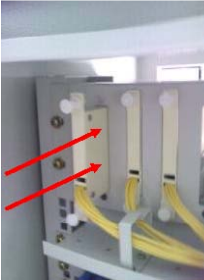
Slot the Splitter Module at the Splitter Slot
