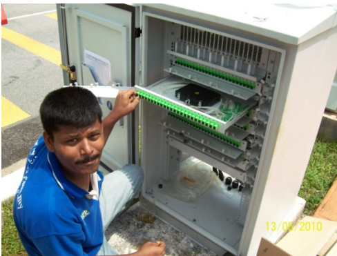
4. Installing adapters
