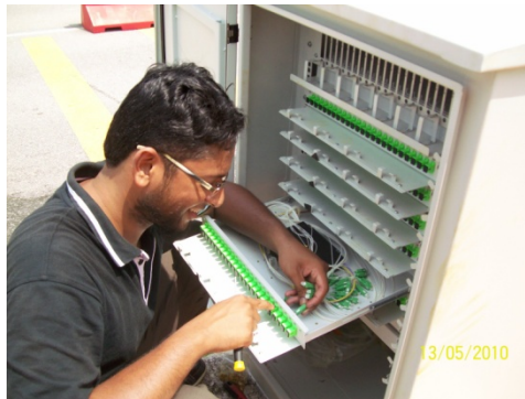
5. Finalizing adapters installation
