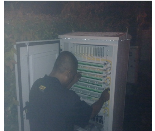
6. Installing splitters
