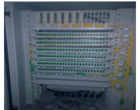
8. After installing splitters
