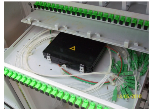
5. Completion of adapter installation
