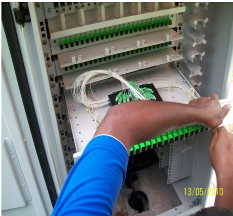
4. Installing adapters
